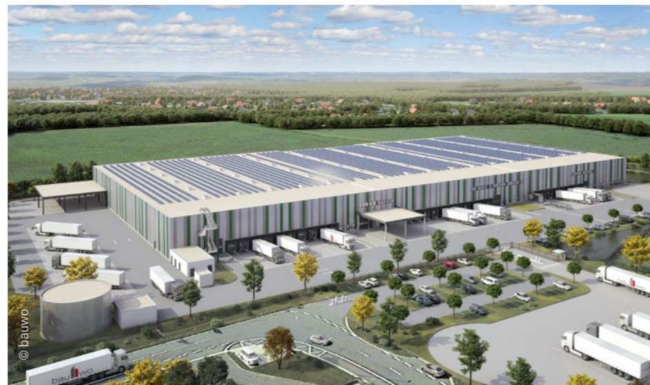
The multiuser logistics facility, which including the mezzanine has around 26,000 square metres of space, is currently being built in Hodenhagen near Hanover (visualisation).
